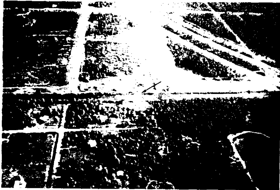
Look north at Golden Gate Weir No. 2 (at arrow). I-75 is at top right.
